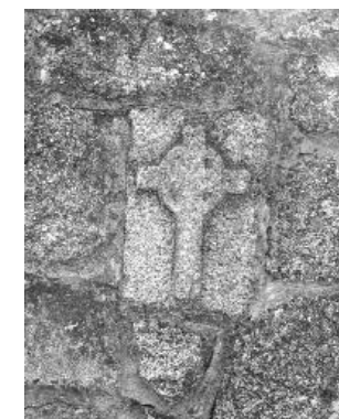
The Celtic Cross on Dalkey Avenue Railway Bridge - April 2008
