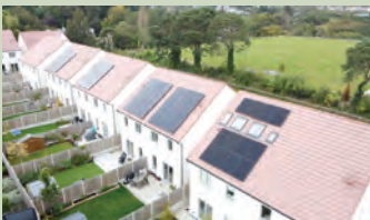
5 roof mounted systems Completed
