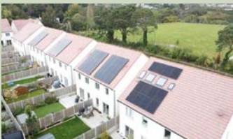
5 roof mounted systems Completed
