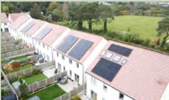
5 roof mounted systems Completed
